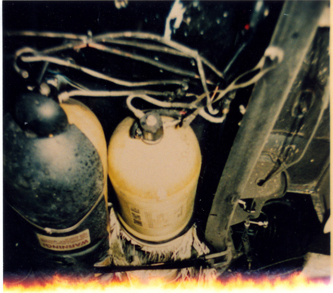
17. Longitudinal View of the Ruptured Cylinder and the Stainless Steel Supply and Delivery Tubing
